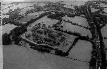
Gloucester's Walham substation is under water
